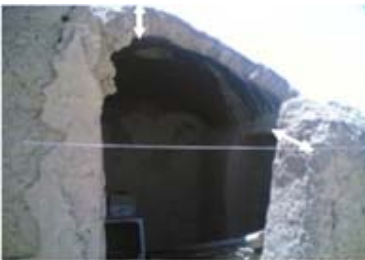
Fig. 3. The thickness of the roof
