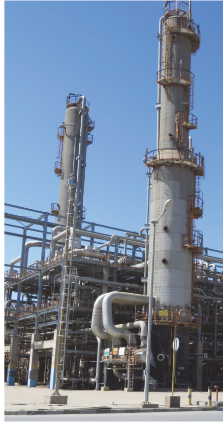
Fig. 3. Abadan Oil Refinery Co Phase 3
