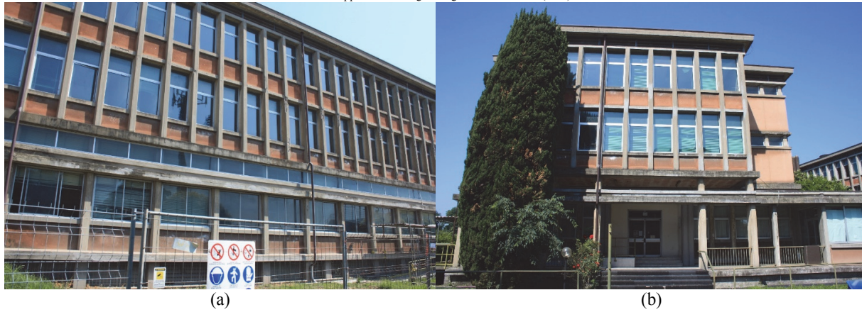
Fig. 3. External view of the building A. Longitudinal façade (a); Main entrance (b).
